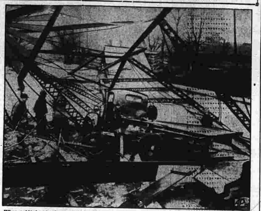
When a 1 1/2 ton truck snapped off the end post of a 120-foot bridge...
